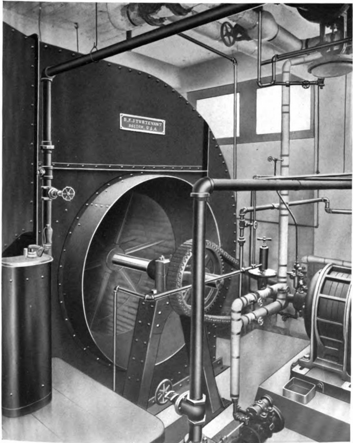
No. 14 MULTIVANE FAN Double Width, Double Inlet, Right Hand, Top Horizontal Discharge Driven by Morse Silent Chain Drive and Induction Motor Heating and Ventilating the Factory of Brown-Lipe-Chapin Company, Syracuse, N. Y.
